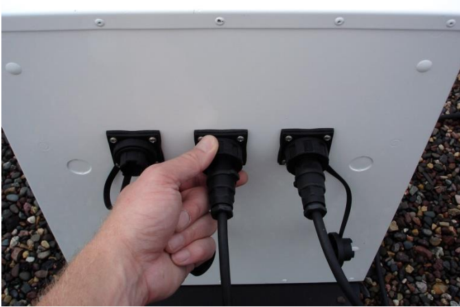
Figure 39: Connect Solar Cells to Battery Enclosure Box
