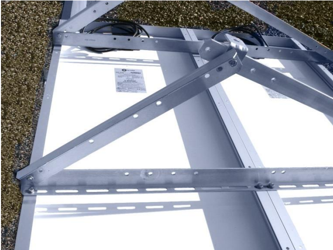
Figure 37: Assemble the Solar Cells on the Mounting Frame
