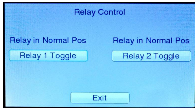
Figure 15. Relay Outputs screen in Diagnostics menu
