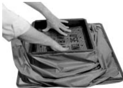
Figure 6: Installation of LoFlow screen
