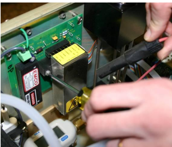
Figure 4. Removing Power Supply
