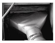
holes and joints, permitted UFPs to enter the basement area. In addition, the vent serving the boy's bedroom was so loose that UFPs had a direct pathway to upstairs living areas.
