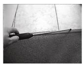
joint directly above the first-floor construction area. Despite careful planning and controls, construction fumes were migrating to the second floor through this unexpected pathway because of a pressure differential between the spaces.
