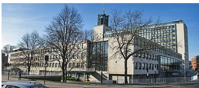
Citation: Sanderson, P., et al. “Characterisation of Iron-Rich Atmospheric Submicrometre Particles in the Roadside Environment.” Atmospheric Environment 140 (2016): 167–175. Photo credit: http://manchesterhistory.net/architecture/1960/civiccentre.html
